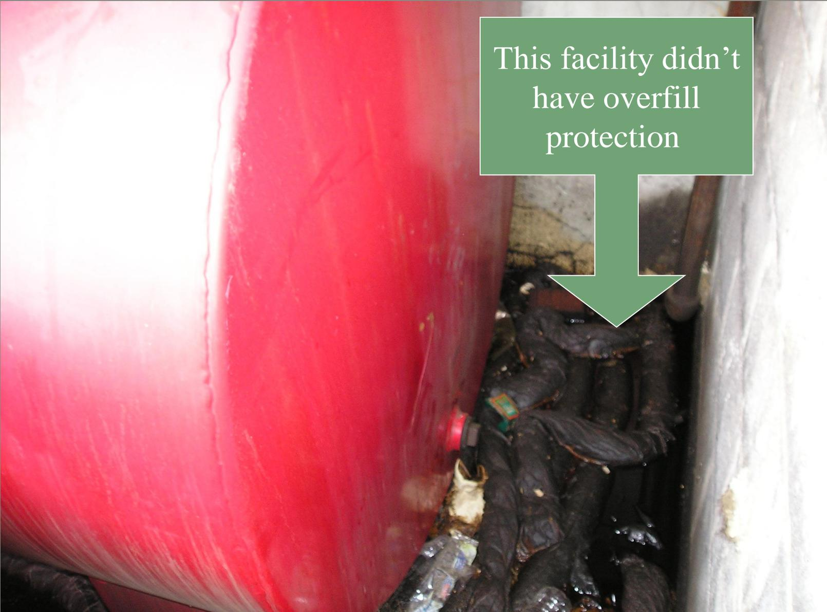
A photograph showing a large red storage tank on the left. To the right of the tank, a dark, viscous liquid has spilled onto the ground, forming a large, dark pool. The spill is contained within a narrow channel between the tank and a white wall or structure. A green arrow points from a text box above down to the spill. The text box contains the text: "This facility didn't have overfill protection".
